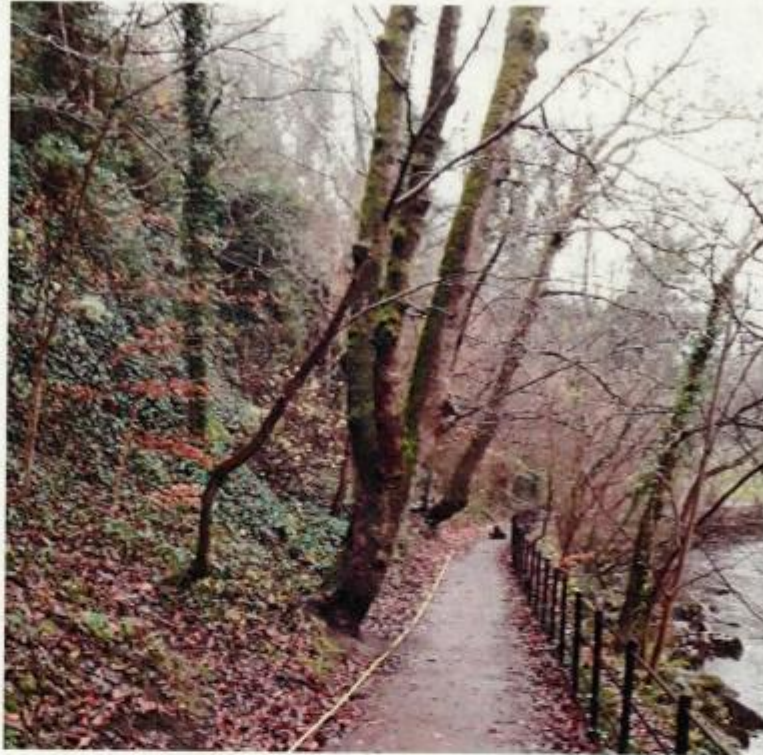
Figure 7a: General view of lower slopes between chainages 90 m and 135 m
