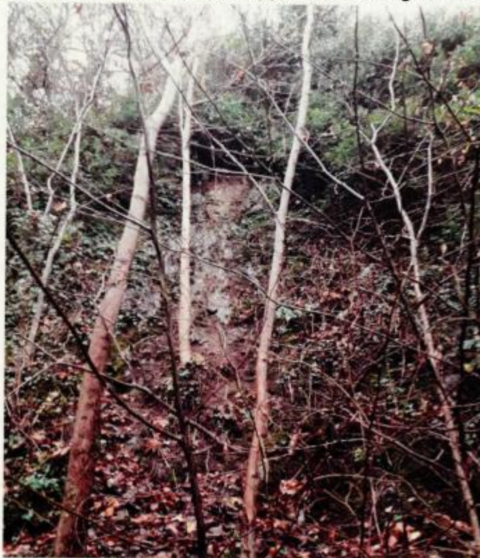
Figure 7b: Recent failure scar on intersecting joints at chainage 115 m
