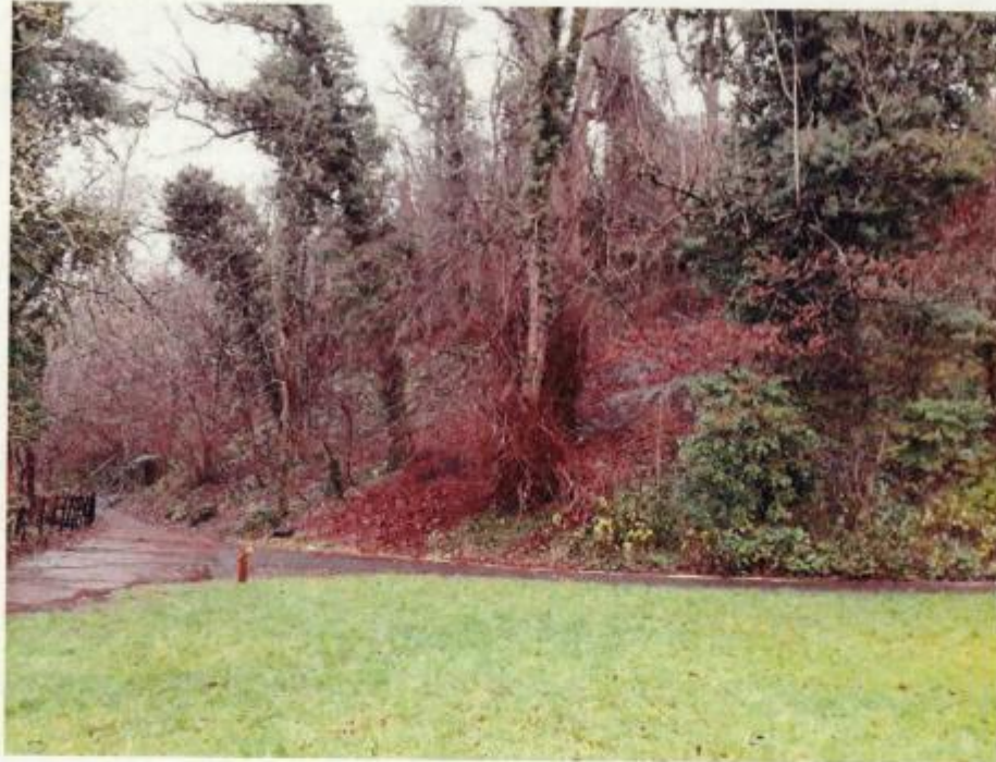
Figure 8b: View of slopes at chainage 170 m
