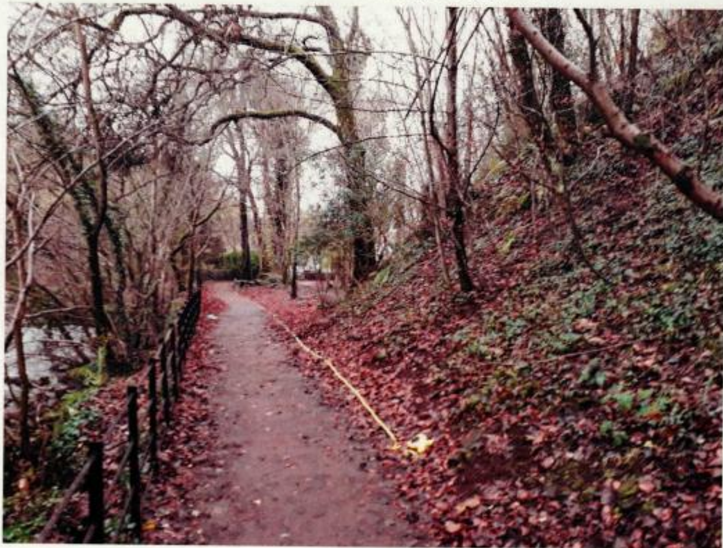
Figure 6a: General view of lower slope at chainages 77 m to 90 m
